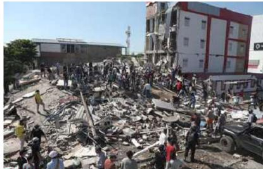
Rattled earth: Residents and rescue workers search through the rubble of a collapsed building in Cali, Colombia, on Monday. AP
